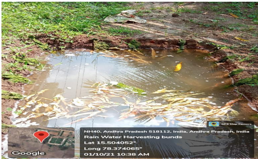
Fig: tanks and bunds
