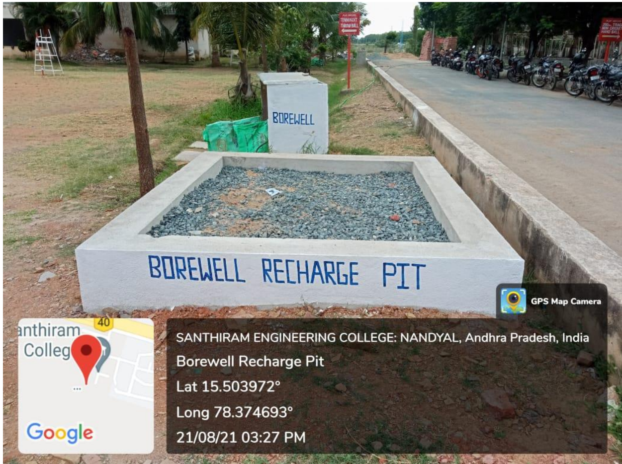
Fig: Bore well Recharge Pit
